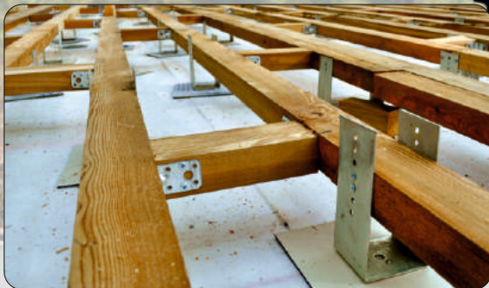
Installation of framework for 1 and 2 floor decking
