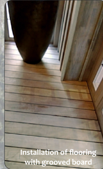
Installation of parquet flooring with teak deck boards
