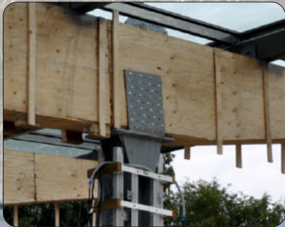
Installation of long LVL roof beams to RUS 360x600x600
